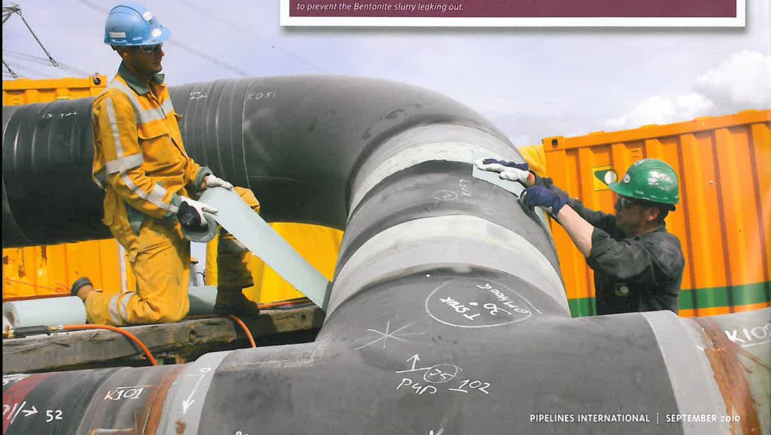
The seal, through which the pipe is thrust, that is used in the launch pit to prevent the Bentonite slurry leaking out.
