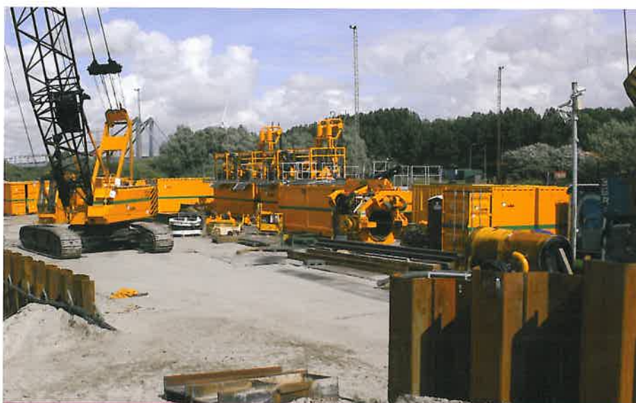
A.Hak's equipment at the worksite.
